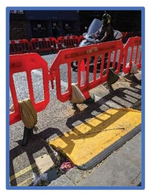
Image depicts an inaccessible pop-up pavementwidening scheme. Barriers have been used to take some of the road space for pedestrians. A temporary ramp has been installed over the kerb, however the space between the ramp and the barrier is too narrow for a wheelchair, mobility scooter or cycle to exit the ramp and turn into the walk way.
