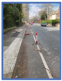
Image depicts a narrow pop-up cycle lane demarcated by a painted white line and bollards. In places nearly half of the width is taken up with mud and debris from trees and two fallen bollards obstruct the path a little further along.
