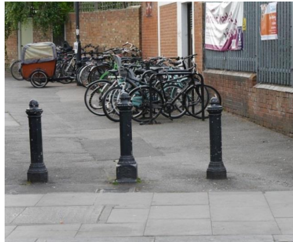
Bollards set closely together, making access difficult or impossible for non-standard cycles
