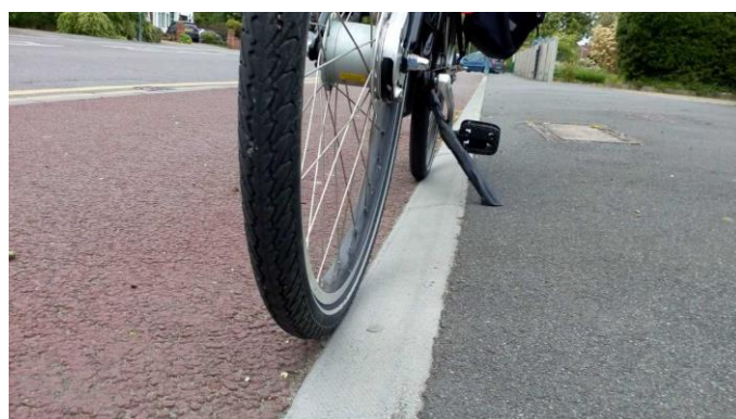
An example of a 'forgiving kerb': a gentle slope allows cyclists to join or leave the track where they like
