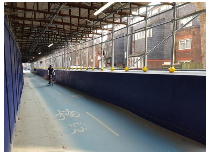
A cycle tunnel has been used here to avoid diversions and the need for cyclists to dismount Credit: TB LCC
