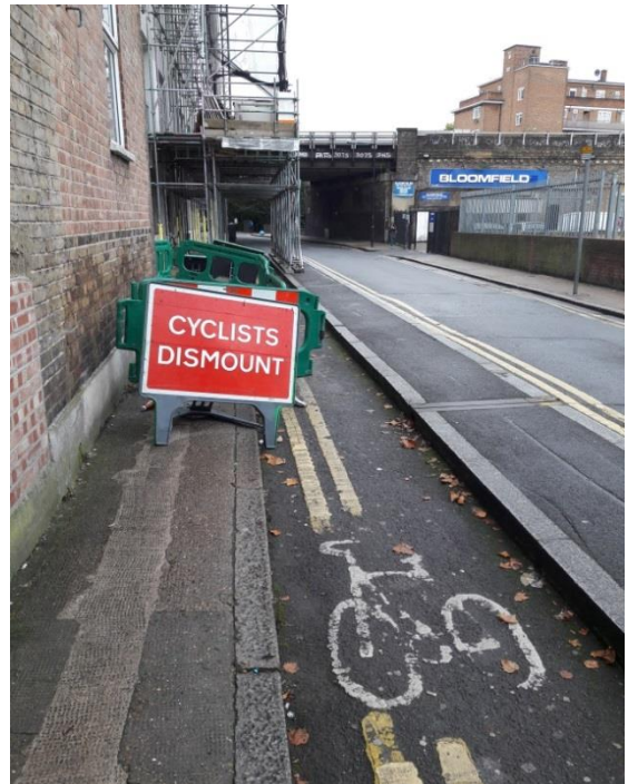
A temporary closure of a cycle lane, which forces cyclists to dismount and lift their cycle onto the island
