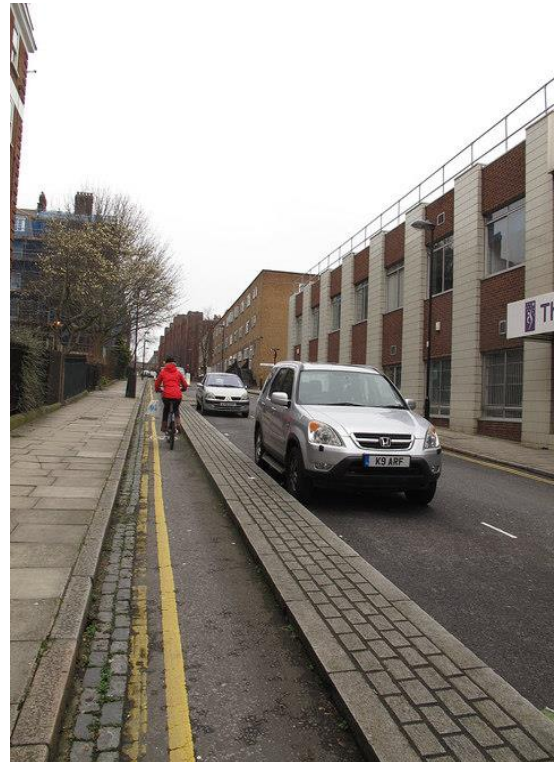
No access to footway and too narrow for many trikes
