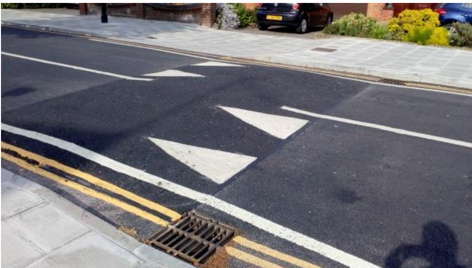
Sinusoidal humps offer the best solution for users of non-standard cycles
