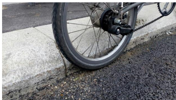
High kerb with no dropped access
