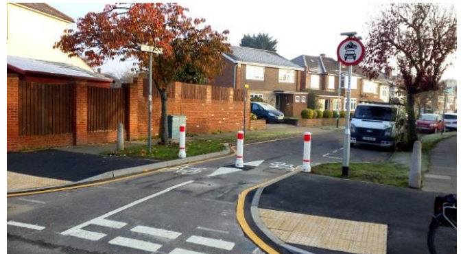
Here there is an air gap of 1.5m between the bollards. Additionally, they have been set into the side road meaning cyclists can complete their turn before going through
