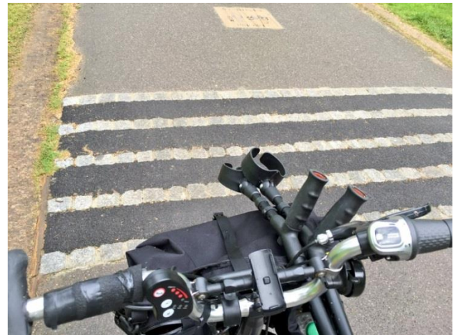
Rumble strips can be painful for cyclists who are unable to stand out of their saddle
